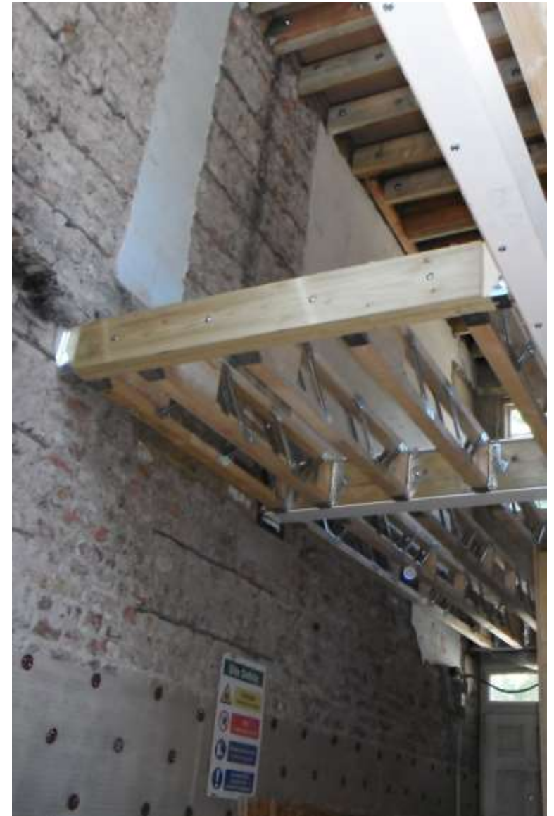
Engineered posi-joist floors
