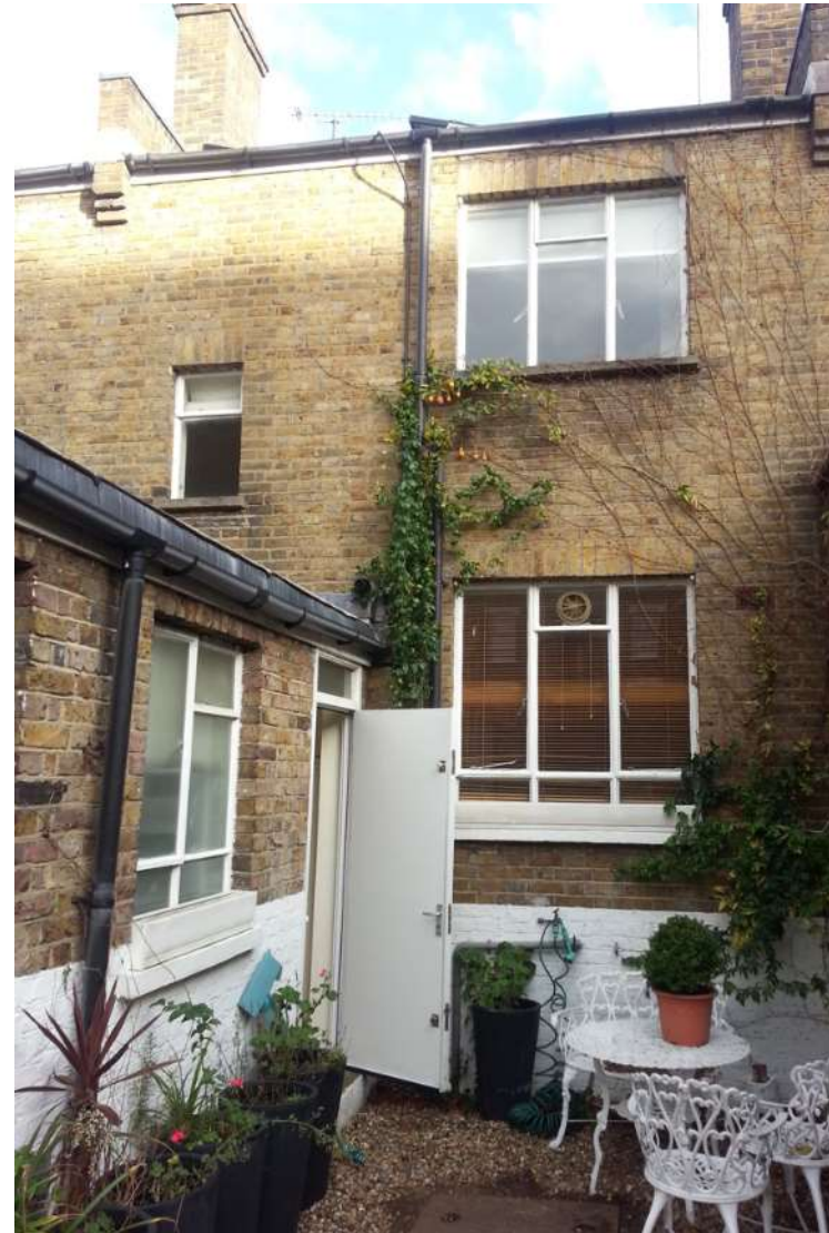
Rear façade with Crittal steel windows
