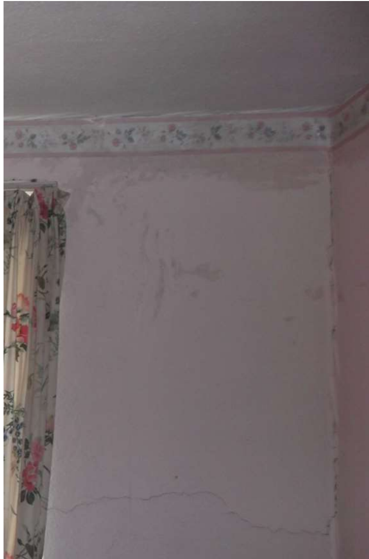
Mould on internal walls
