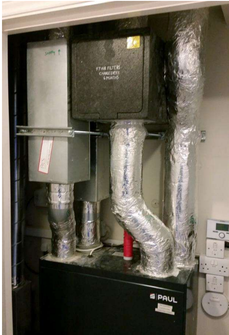
High-efficiency MVHR from Paul + insulated ducts
