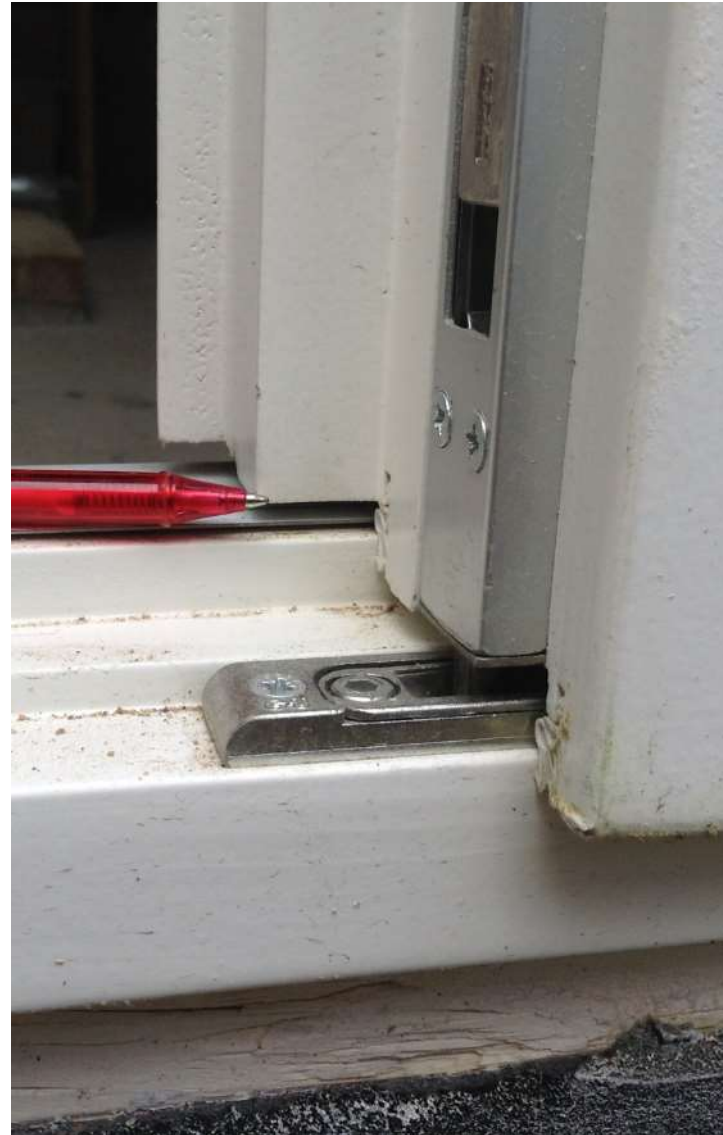
Patio door missing a seal
