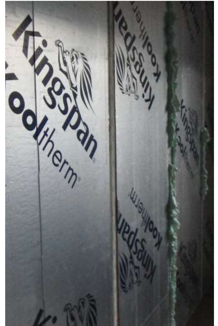
Kingspan in new party walls (foam insulation to all gaps)
