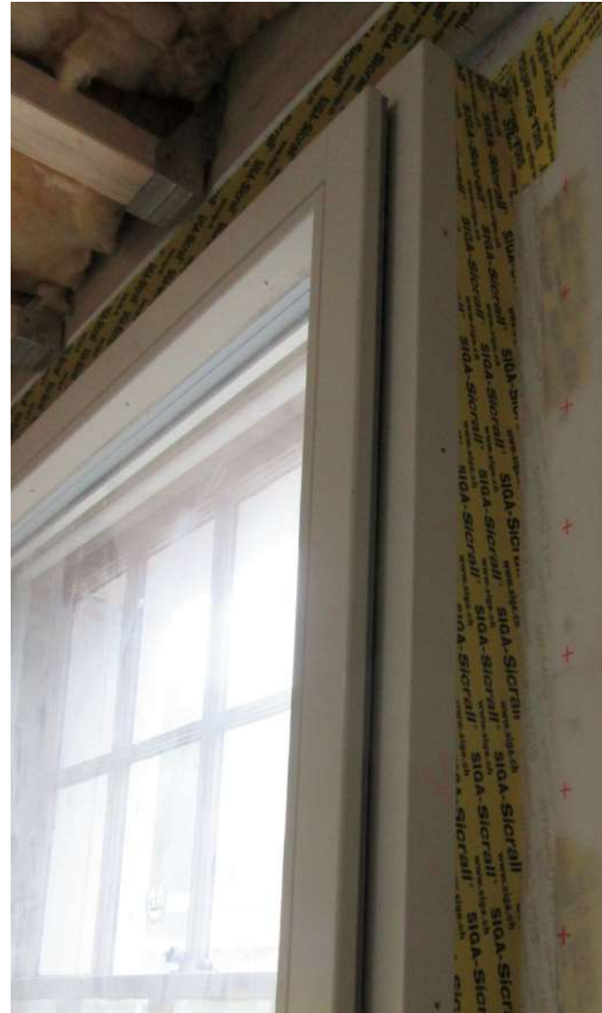
Taped to become airtight
