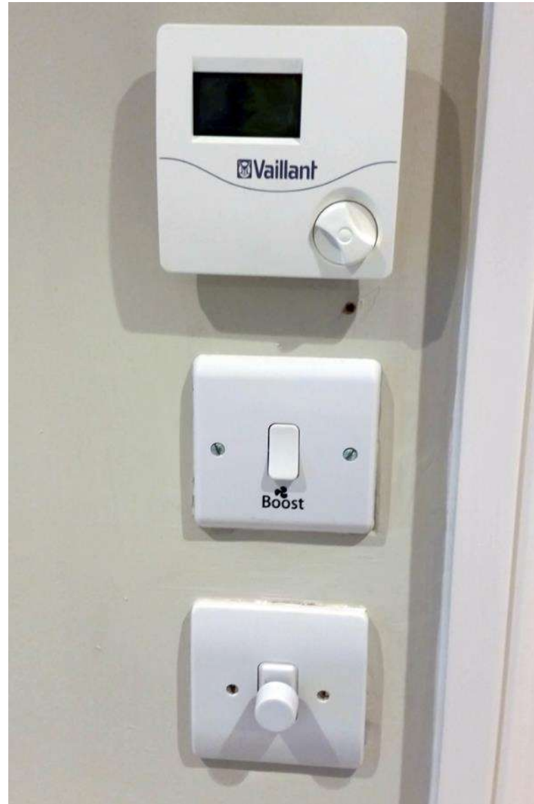
Controls are kept simple, i.e. one boost button for MVHR
