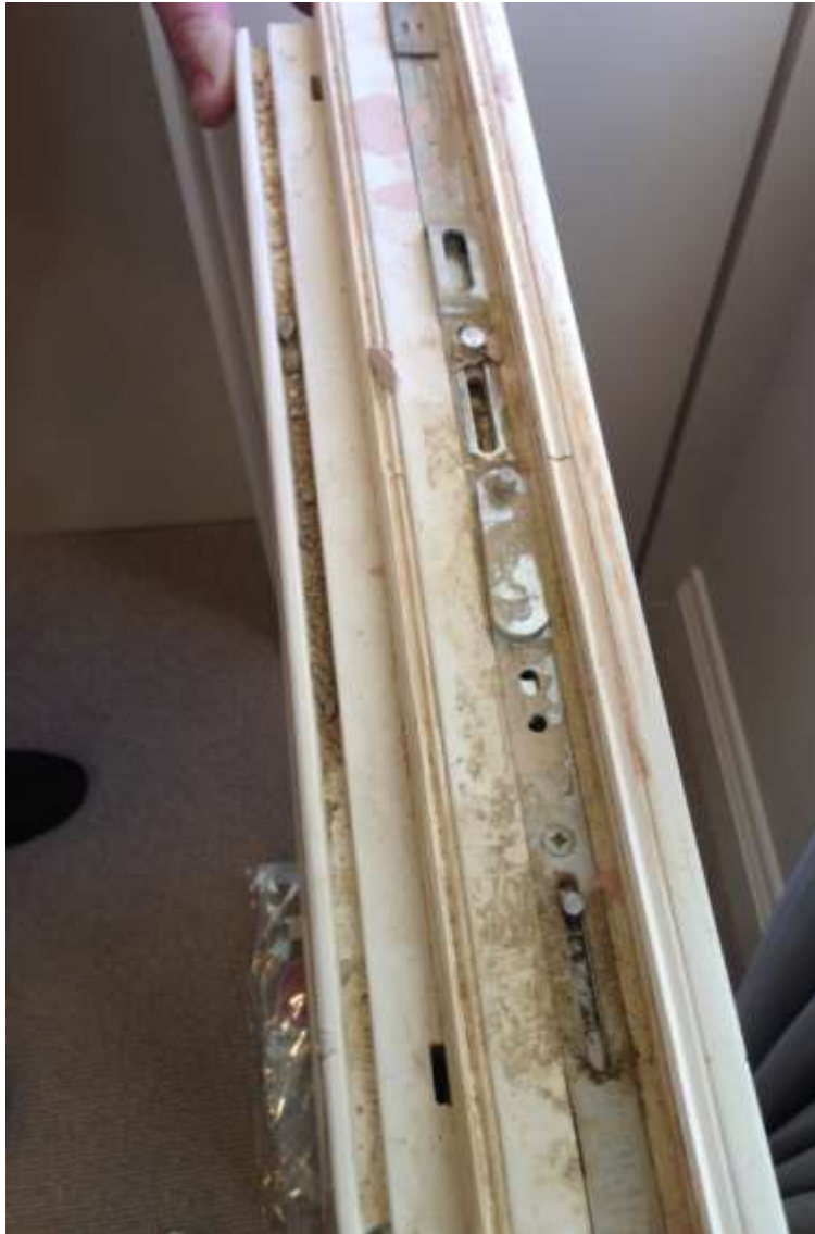
Casement mechanism full of site dirt/ plaster
