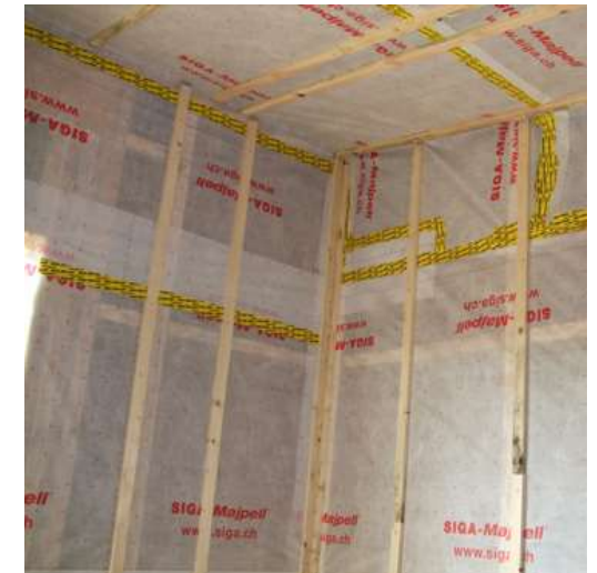
Intelligent membrane – one directional moisture transfer
