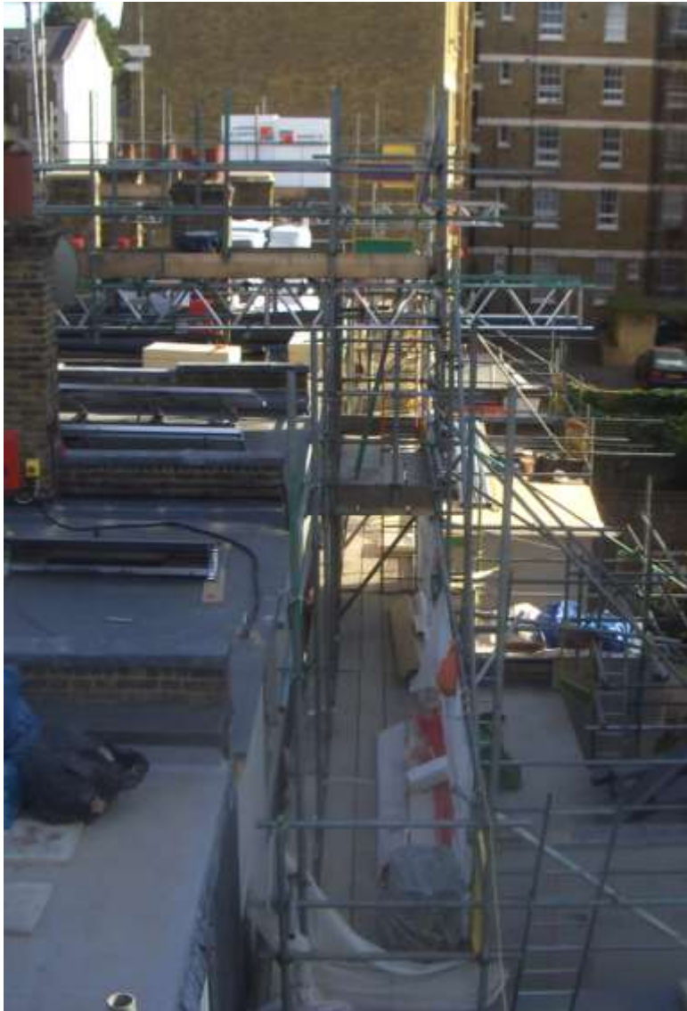
External insulation applied to the whole street
