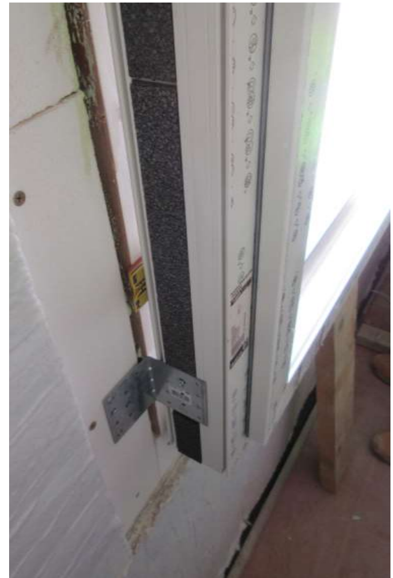
Compacfoam instead of timber support
