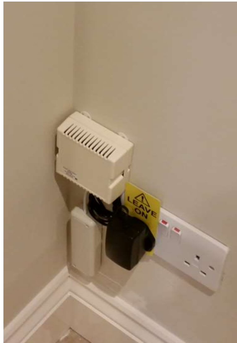
Internal temperature and CO2 meter
