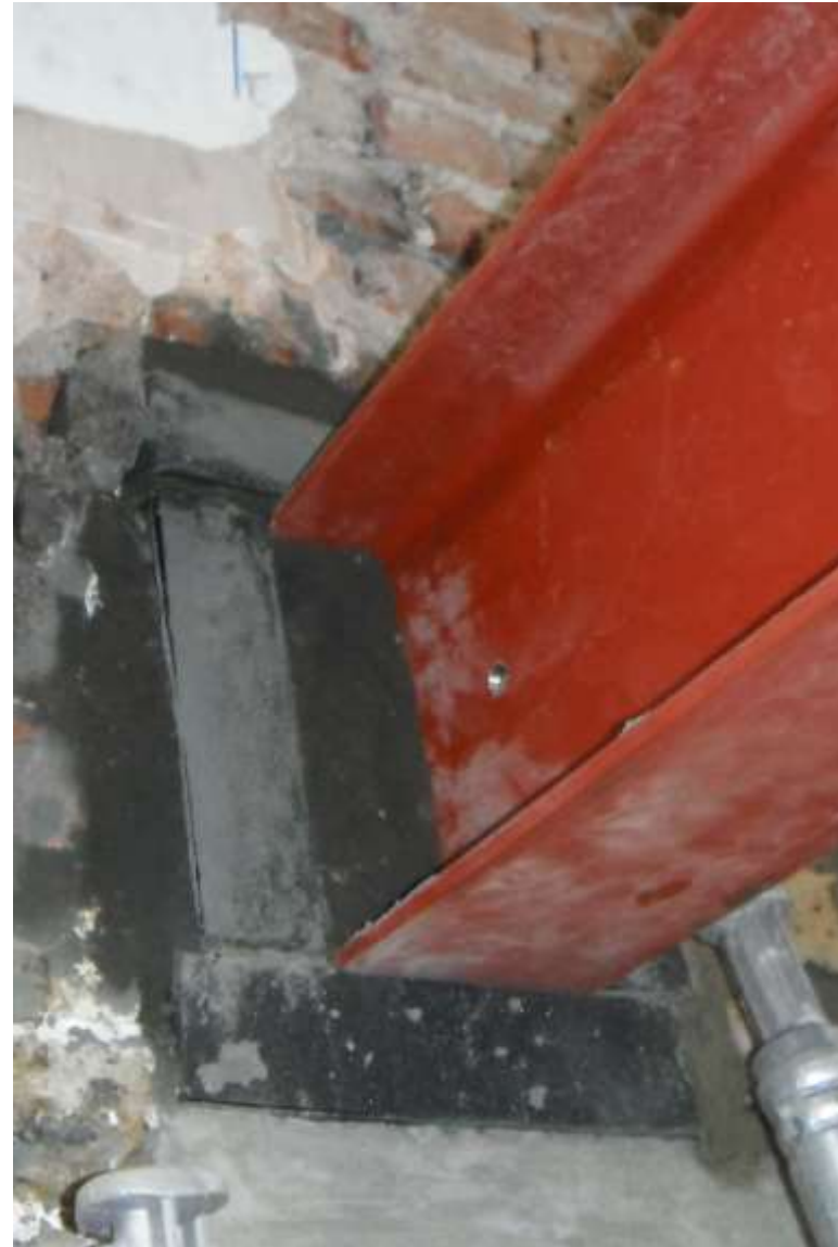
Foamglas cellular glass insulation to steel beams
