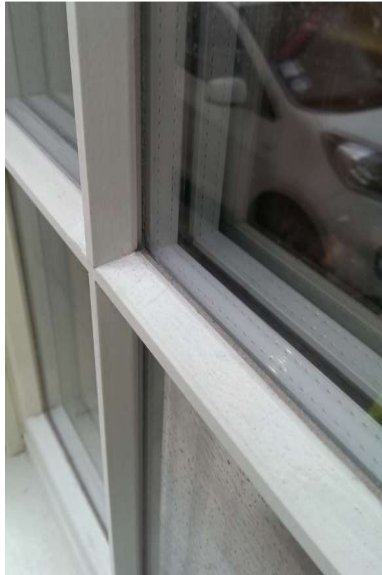
Cold bridging through aluminium spacers
