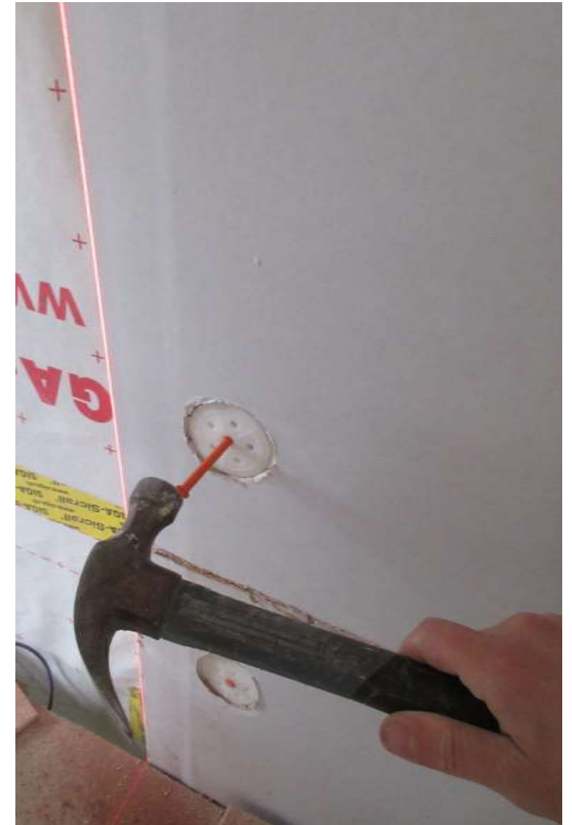
Kingspan in extension and party walls
