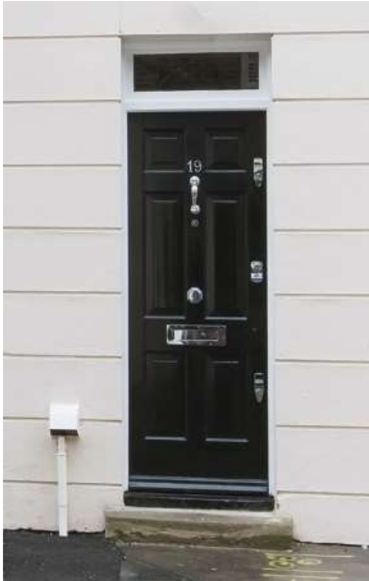
Existing front door
