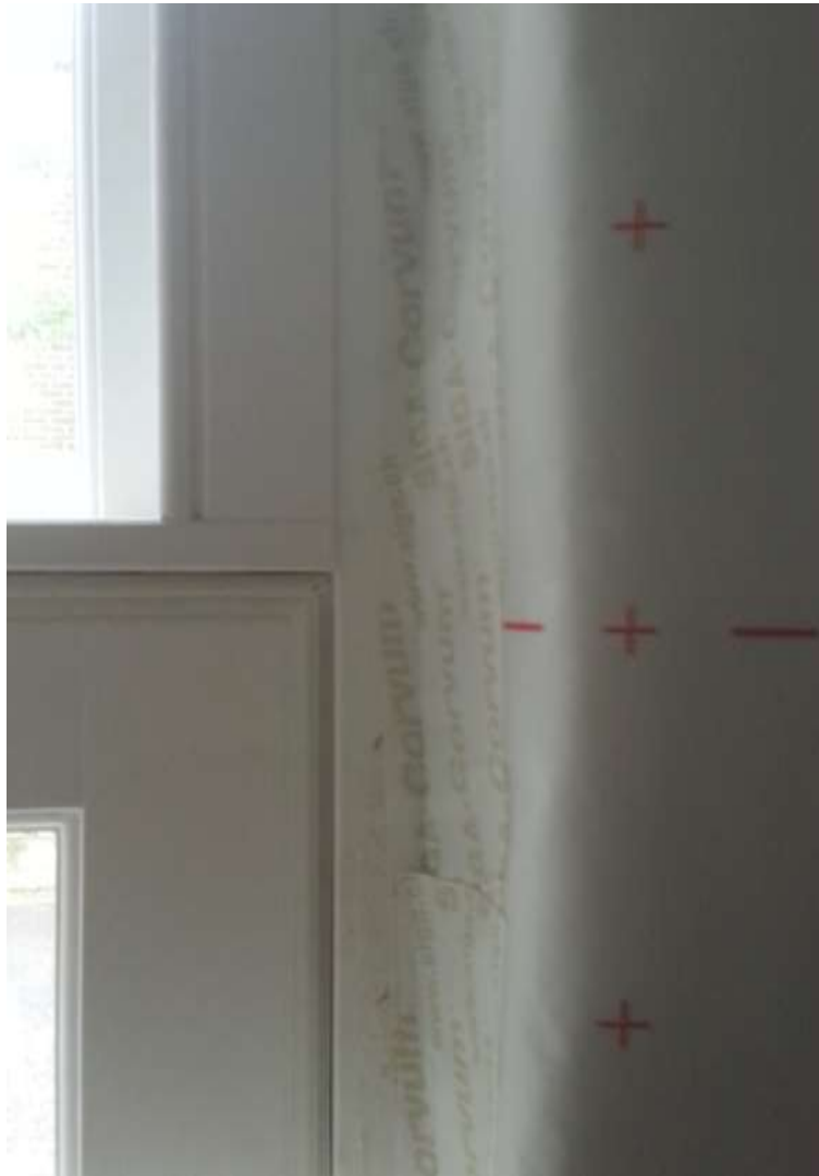
Airtightness tape over window frame
