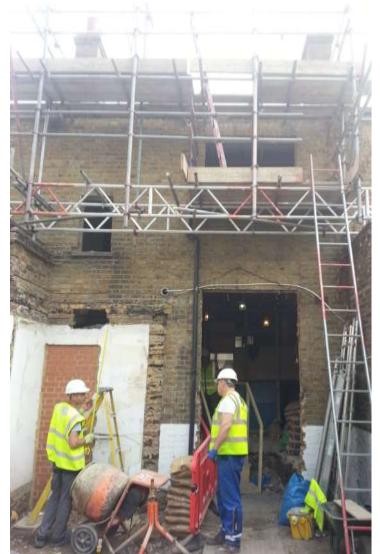
Rear façade retained after demolition of extension
