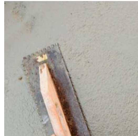
Lime parge coat – acts as a moisture buffer
