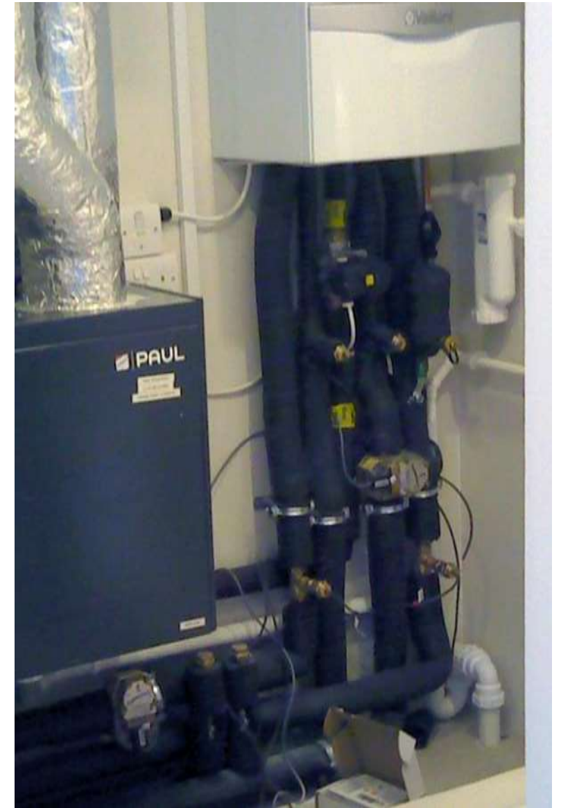
High-efficiency boiler from Vaillant + insulated DHW pipework
