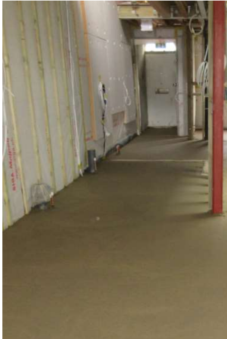
Kingspan insulated plasterboard to party walls
