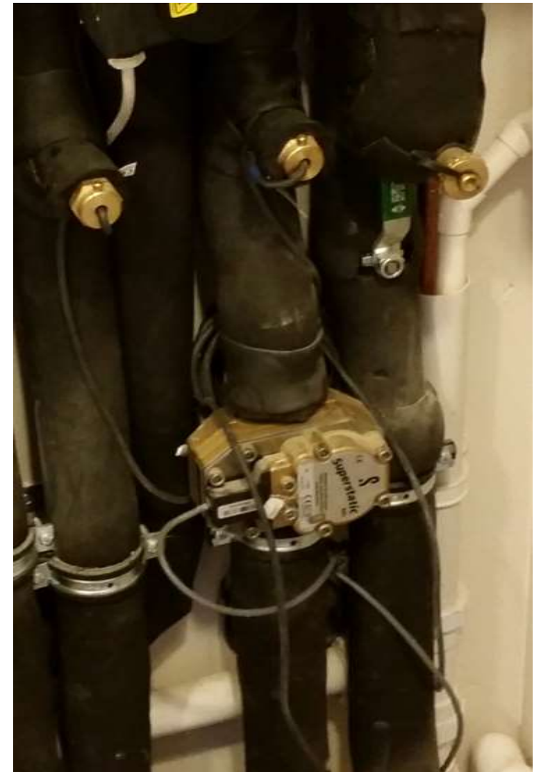
Domestic hot water flux meter
