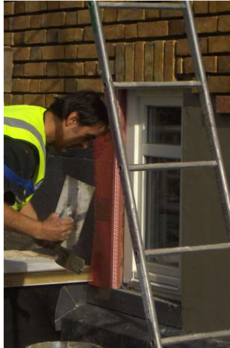
Insulation over window frame
