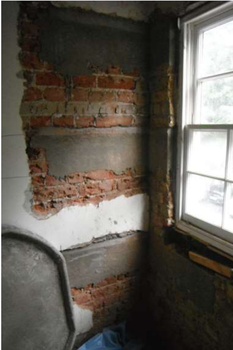
Concrete elbow ties
