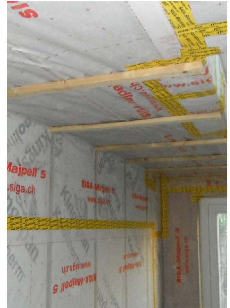
Continuous airtight intelligent membrane
