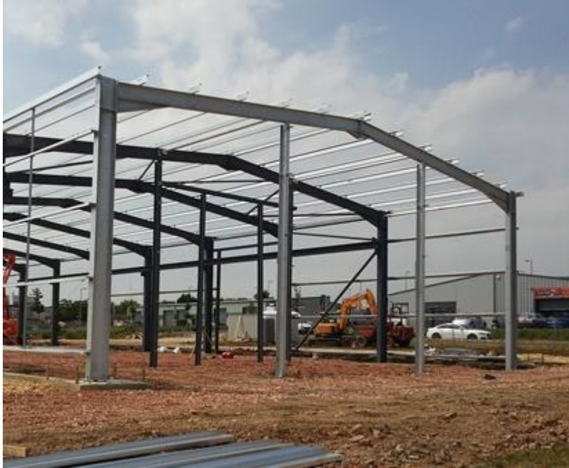
Typical metal portal structure
