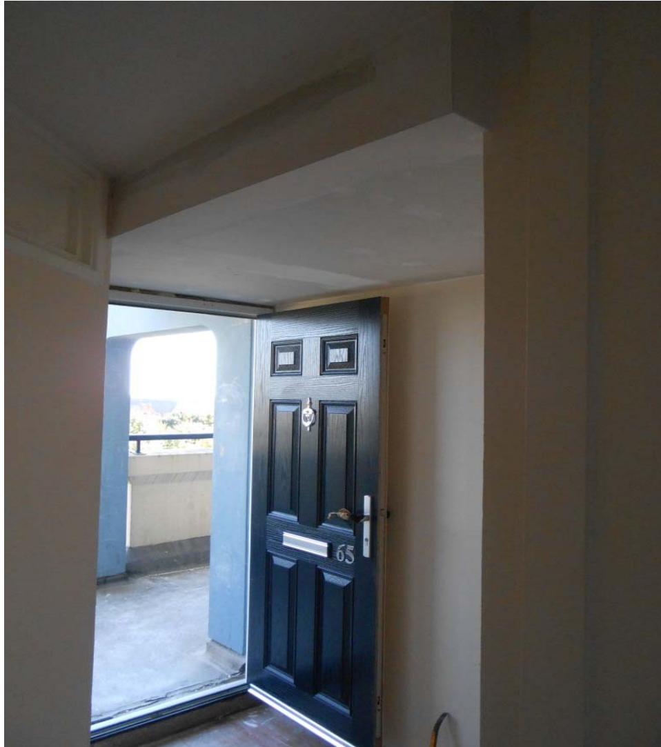
New entrance door and lowered ceiling for exhaust and intake ducting
