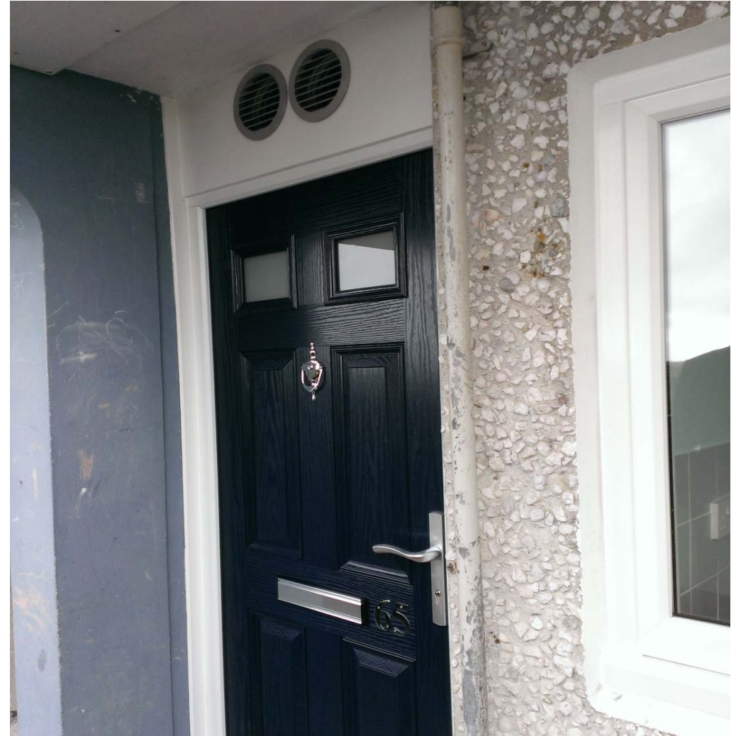
Temporary exhaust and intake valves to corridor. After enclosing the walkways these will be extended to the external wall
