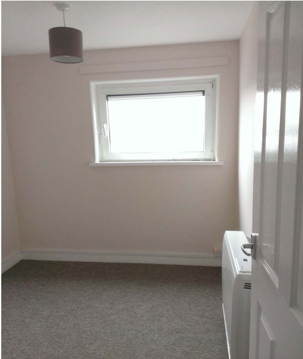
New storage heater in bedroom
