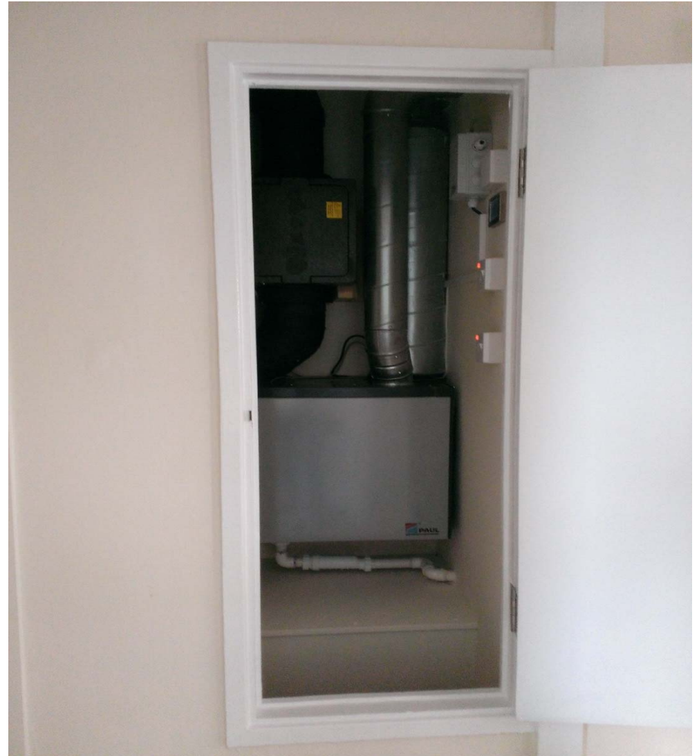
Paul Focus 200 installed and running
