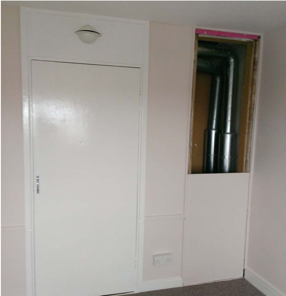
Supply valve in bedroom and ducts in existing riser
