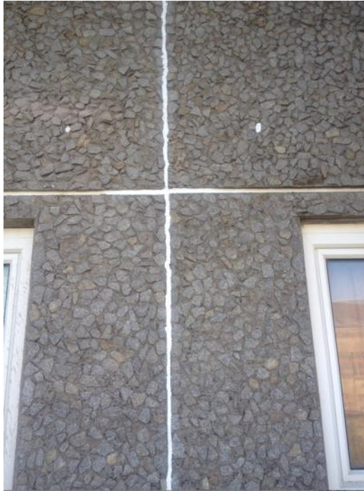
Airtightness jointing – Precast panels
