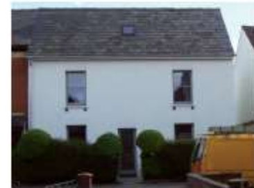
Front elevation post-retrofit
