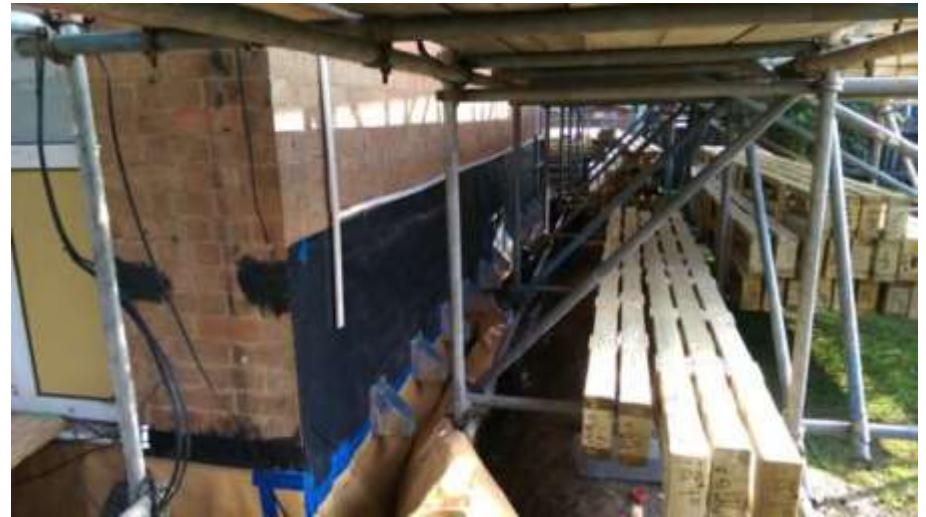
Monarflex DPM fitted to the base of the building
