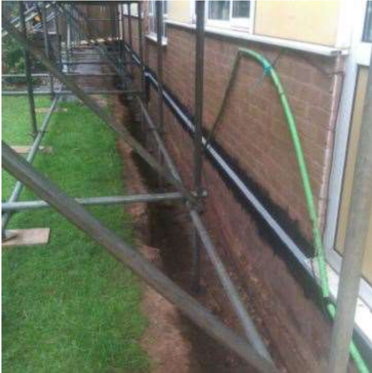
Monarflex DPM fitted to the base of the building
