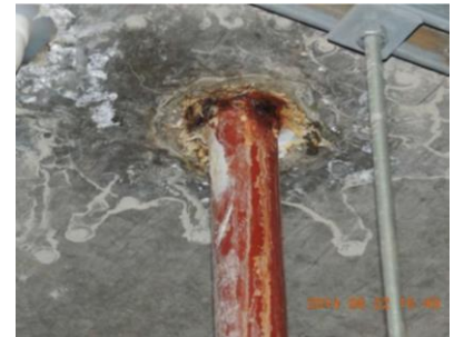
Gas & services leaks
