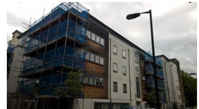
Water penetration through cladding and balconies (leaks)
