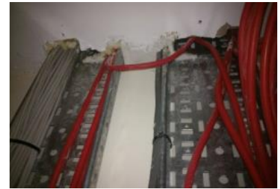
Lack of fire protection
