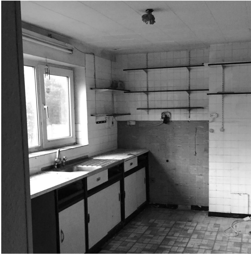
All services to be fully upgraded
