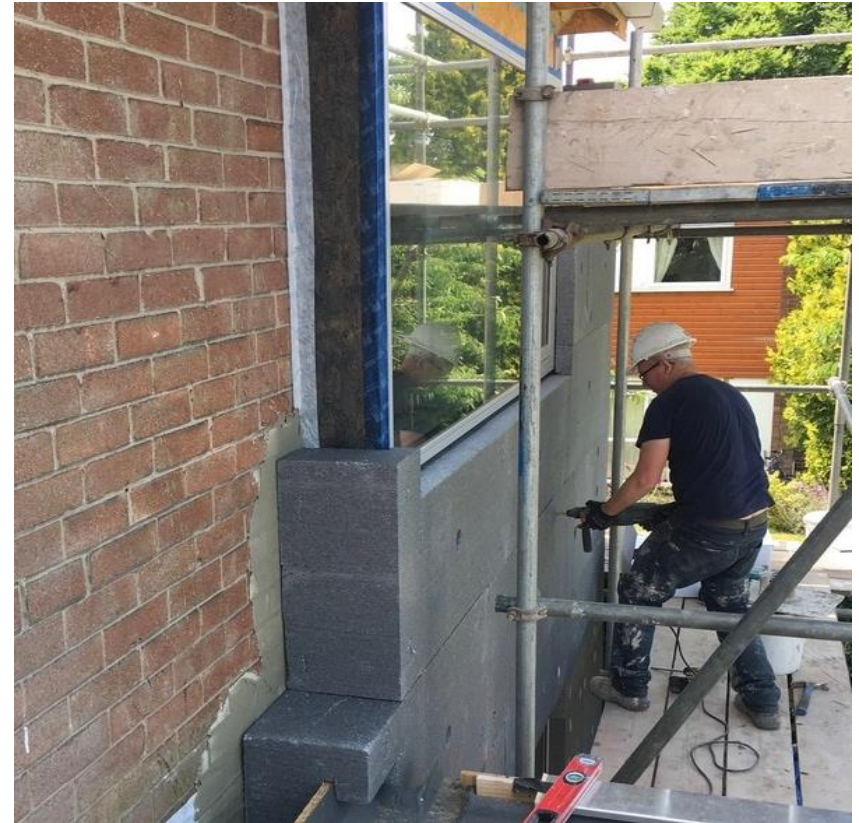
EWI (+ experienced sub-contractor)
