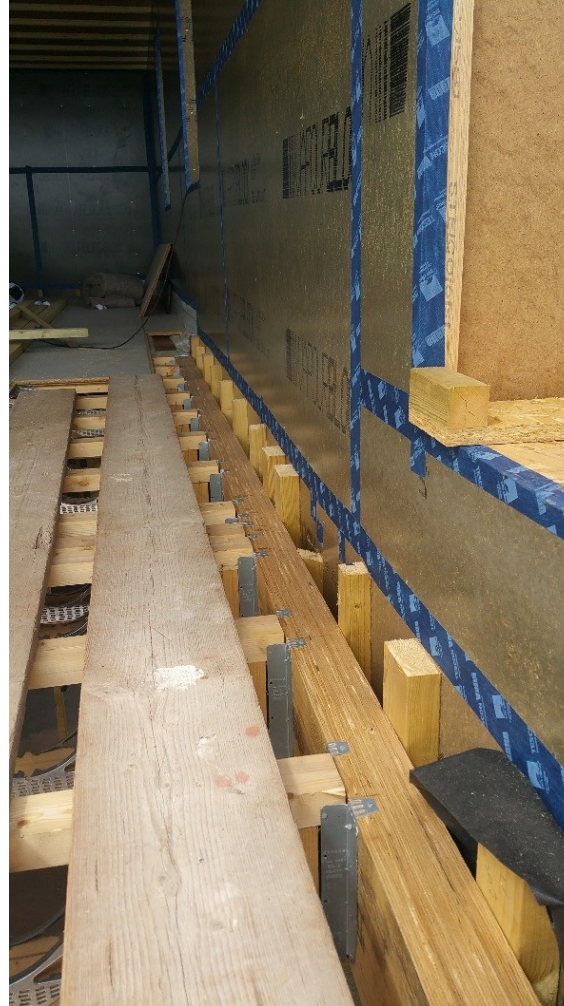
Intermediate floor detail, example of an eliminated linear thermal bridge
