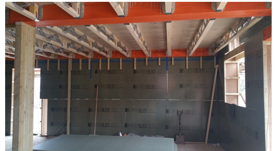
Intermediate floor detail, example of an eliminated linear thermal bridge
