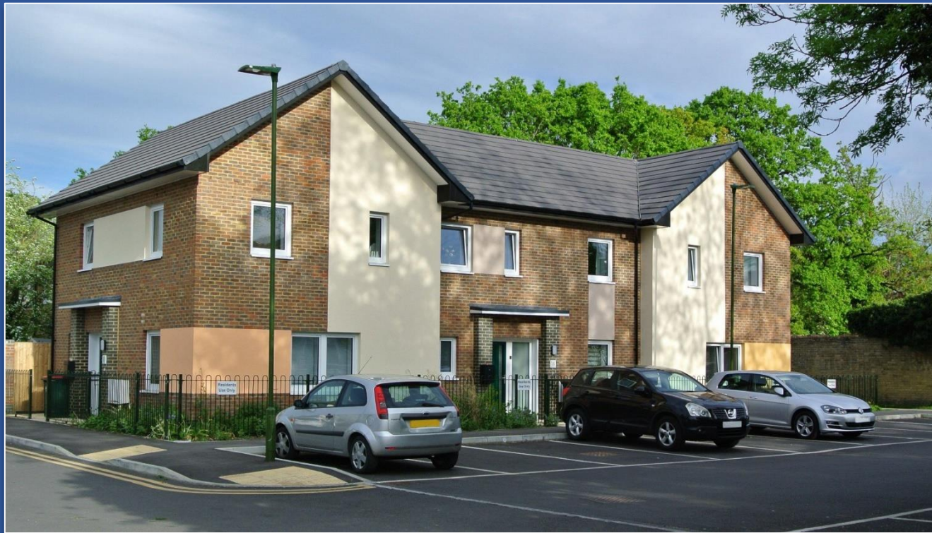
Gales Place, Crawley – certified 2017
