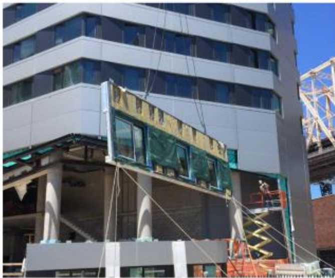
Prefabricated metal wall panel installation
