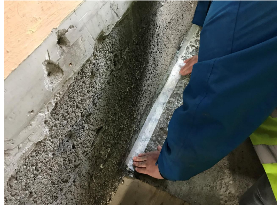
Taped floor to wall junction sealing
