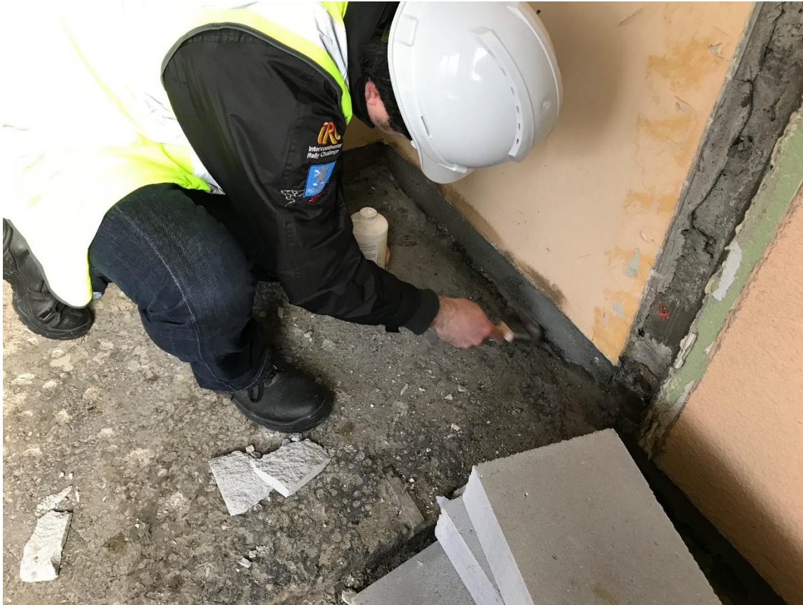
Liquid-applied floor to wall junction sealing
