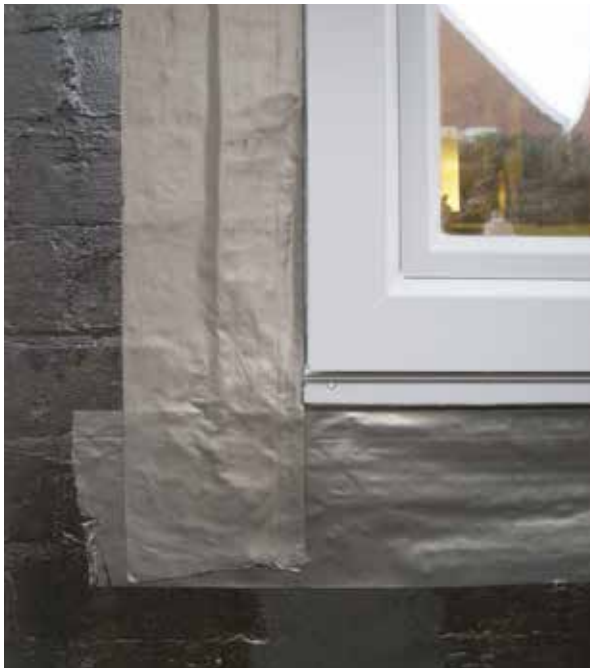
Careful detailing was an essential part of the building's success with tape used to ensure difficult junctions remained air-tight
