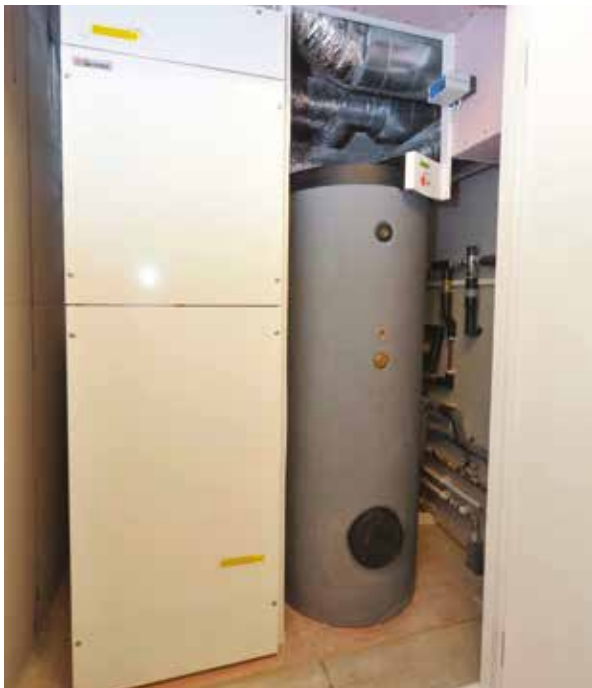
An MVHR unit, fitted within the basement, is the primary source of both heating and ventilation within the property
