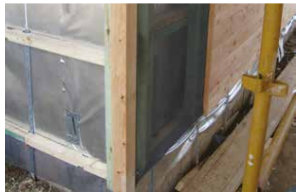
A breather membrane was used as part of the roof build-up to provide an extra layer of water proofing
