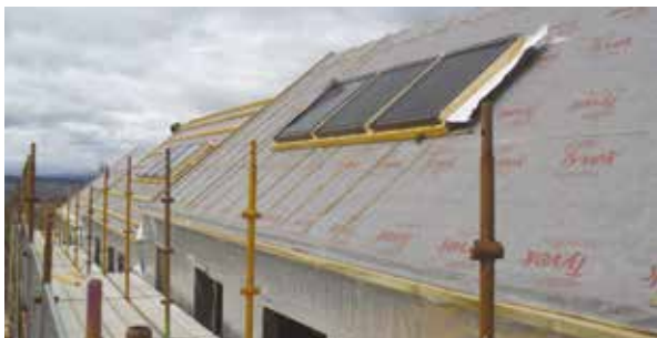
Rooflights were installed on the terraces to maximise solar gains helping to reduce heating bills (Image courtesy of HLM Architects)
