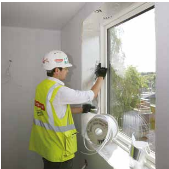
Careful detailing was used to ensure thermal performance and air-tightness with Kingspan Thermawall ® TW55 cut to insulate around the windows and tape used to improve air-tightness (Image courtesy of Shepherd Construction)
