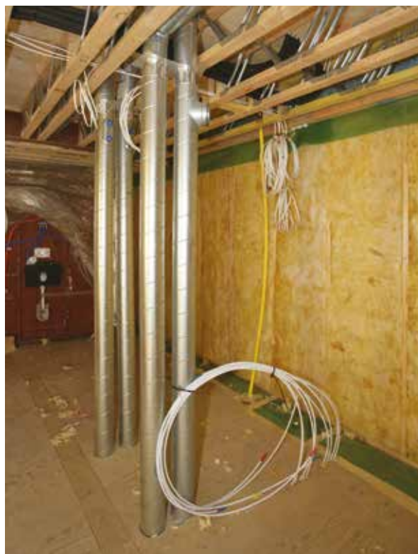
In order to keep the living space uncluttered, ventilation ductwork was largely concealed within the walls and ceilings (Image courtesy of Shepherd Construction)
