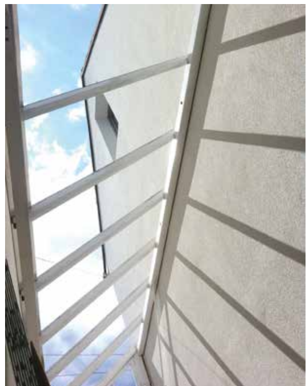
The new extension used extra glazing to maximise solar thermal gain within the building, minimising heating usage
