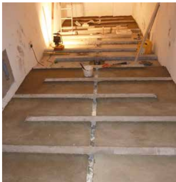
A labyrinthian heat exchanger was fitted under the basement floor, using the more constant temperature of the ground to provide cooling in the summer and pre-heating in the winter
