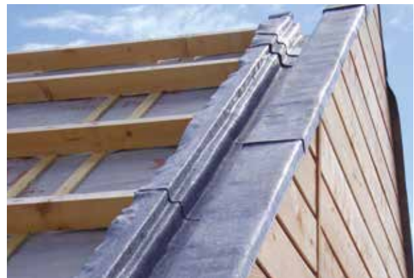
A breather membrane was used as part of the roof build-up to provide an extra layer of water proofing
