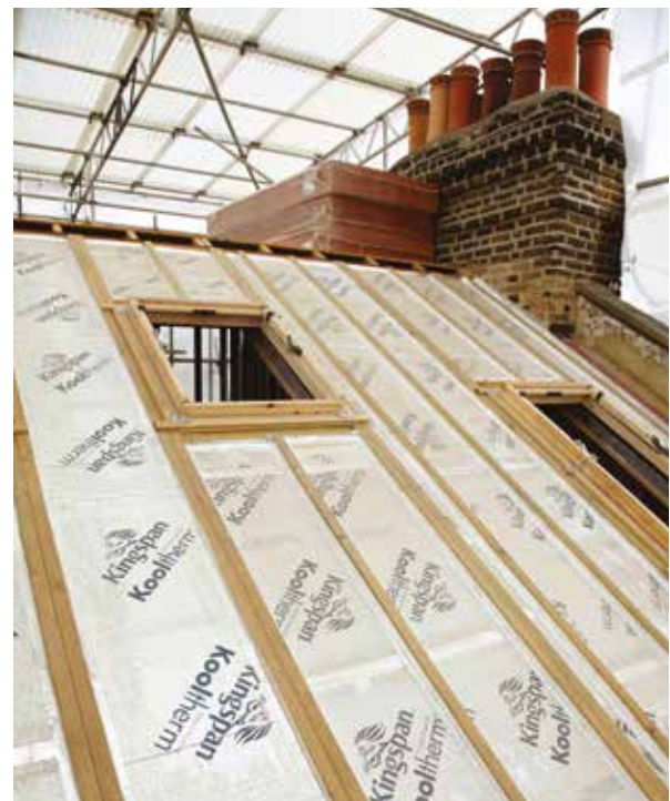
130 mm of Kingspan Kooltherm ®, fitted between the roof rafters, provided the first layer of insulation to the roof of the property
