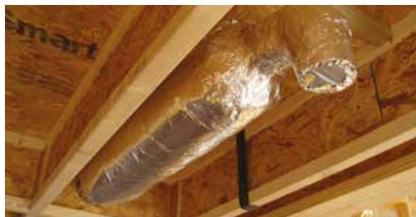
Ventilation ductwork was concealed within roof and wall space and OSB board used to minimise air-loss (Image courtesy of HLM Architects)
