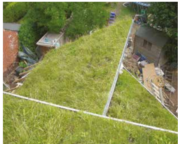
The roof of the new rear extension was specially built to be covered in green roofing
