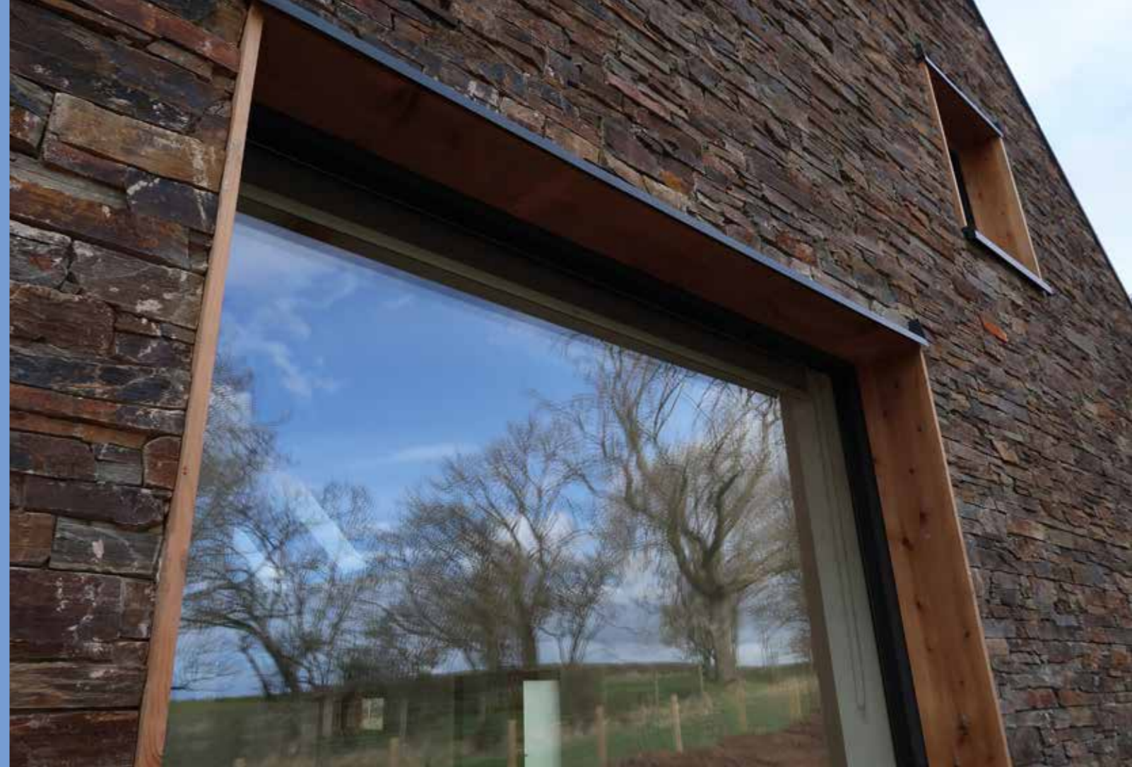
LOCH LEVEN LOW ENERGY NEWBUILD cover: FISHLEYS PASSIVHAUS
