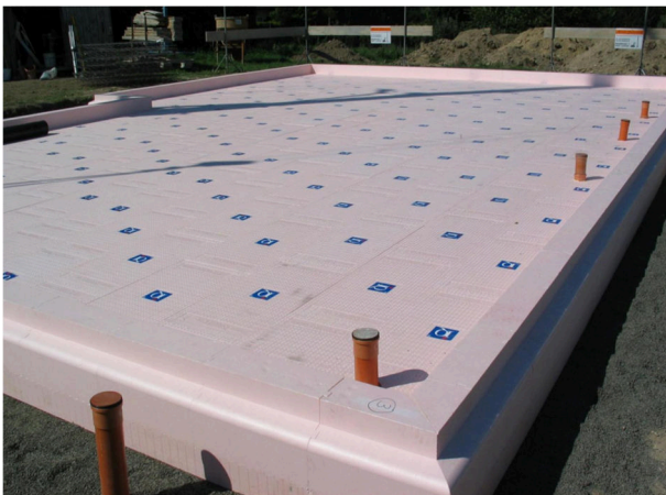
Diagram 5 - typical System installation prior to installation of DPM
