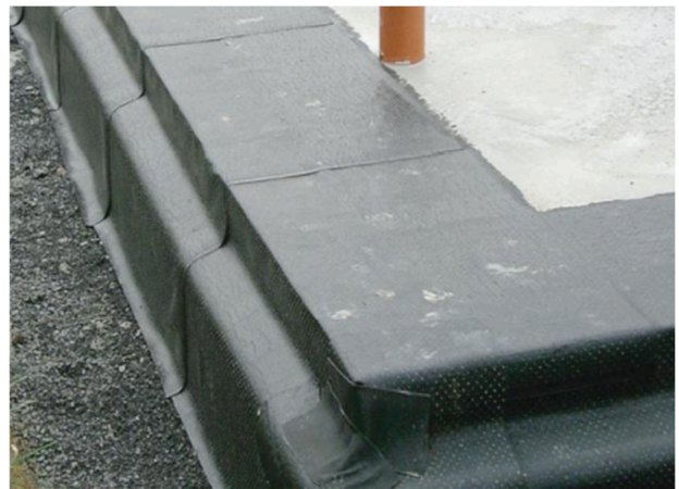
Diagram 6 - typical installation of System edge protection
